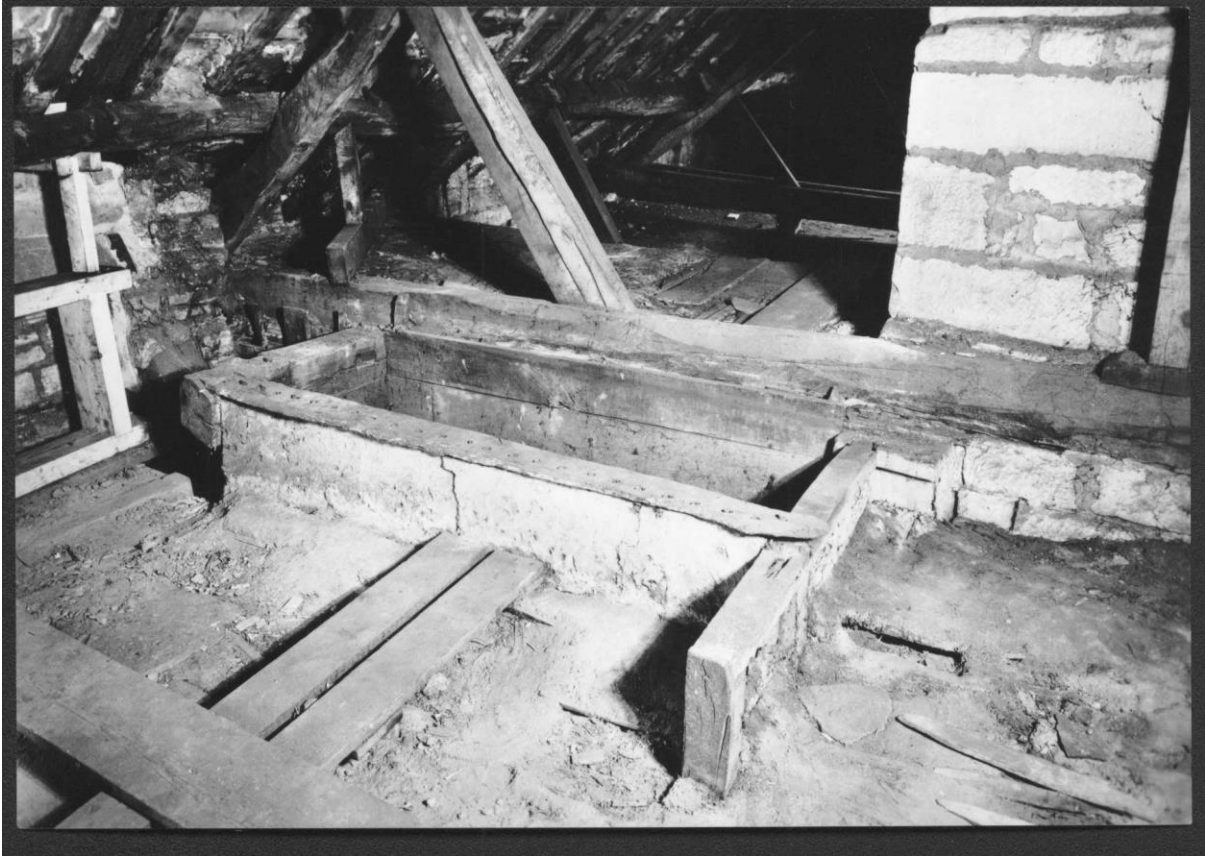
Hall I' th' Wood attic space
